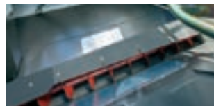
Smooth surfaces in the grain tank
