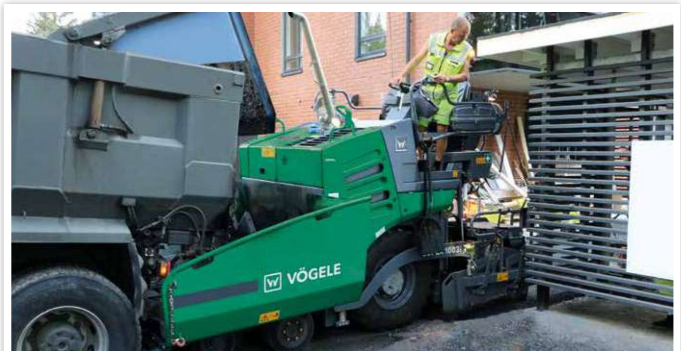
REHABILITATING ACCESS ROADS
