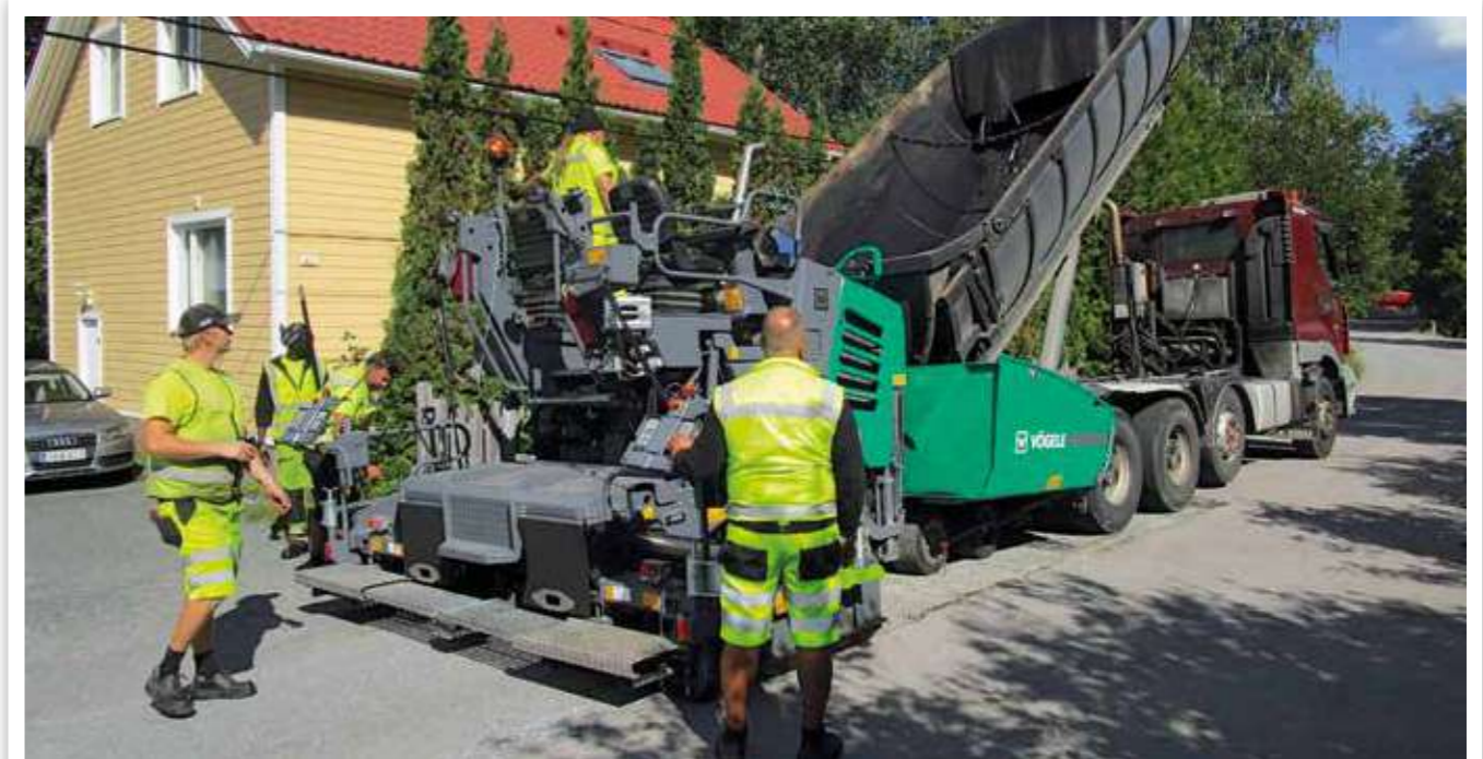
PAVEMENT REHABILITATION ON MUNICIPAL ROADS
