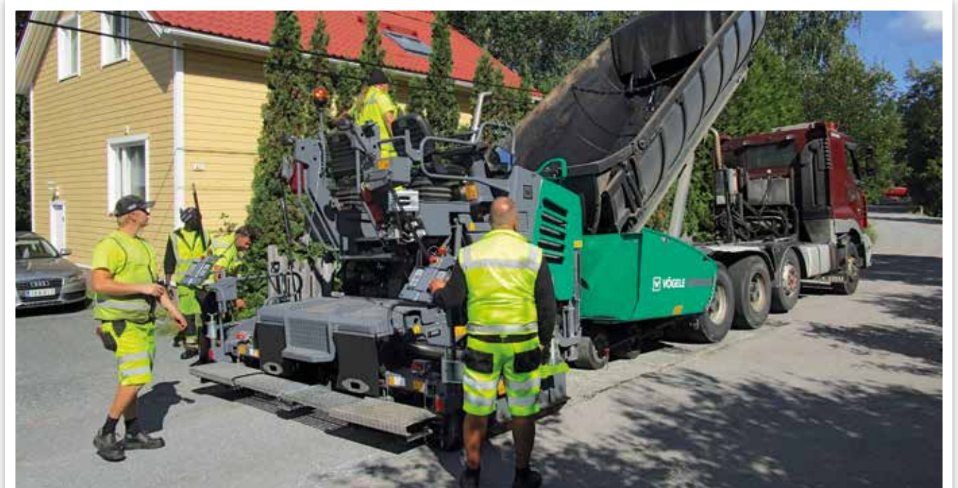
PAVEMENT REHABILITATION ON MUNICIPAL ROADS
