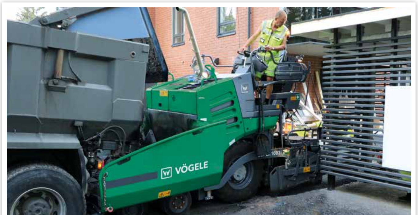
REHABILITATING ACCESS ROADS
