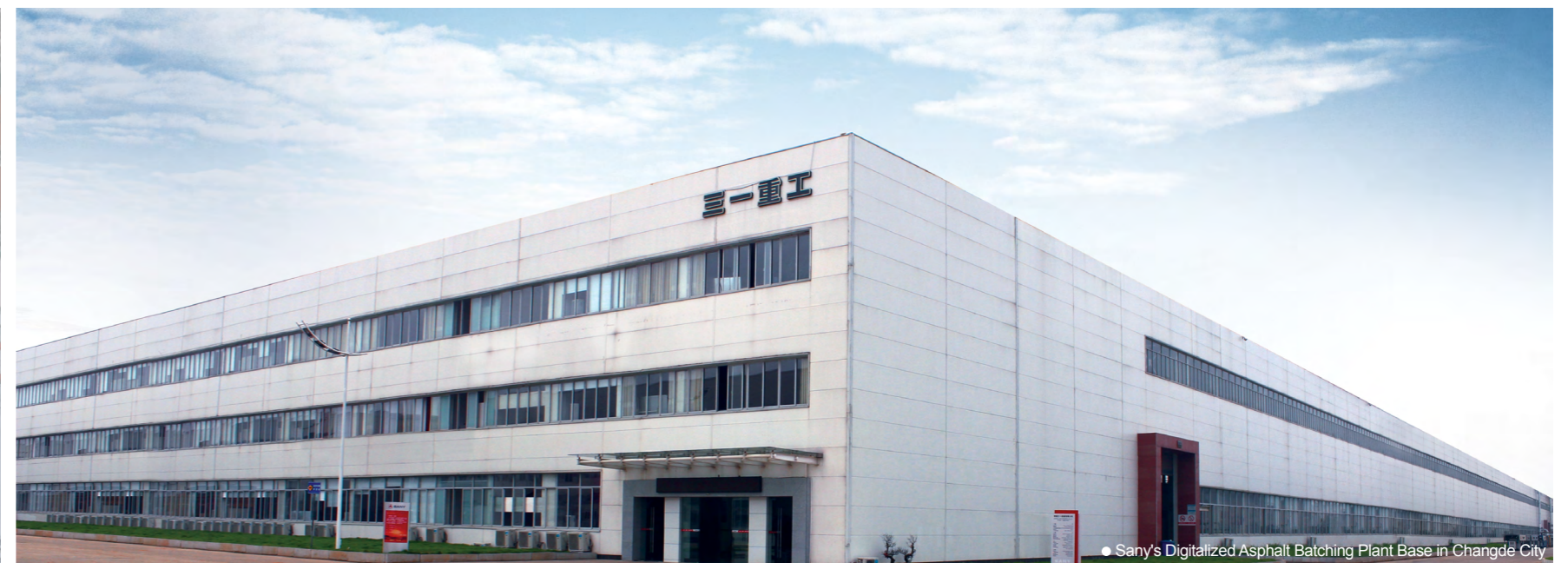
● Sany's Digitalized Asphalt Batching Plant Base in Changde City
