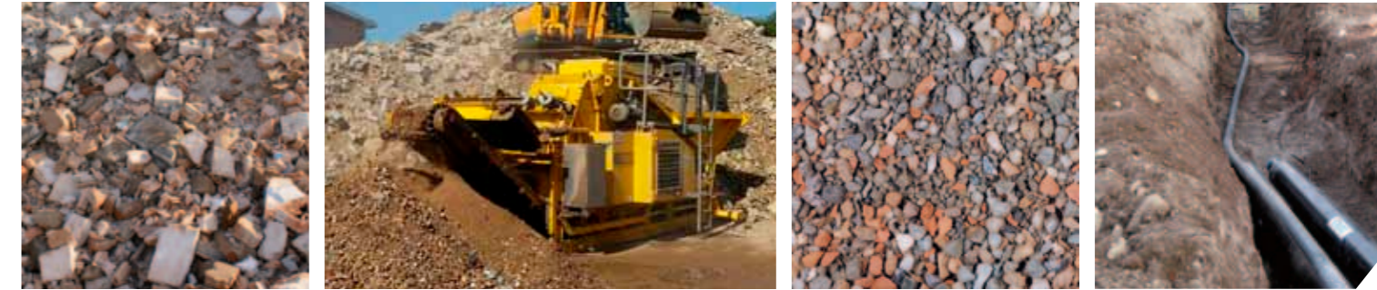
Rubble Processing Recycling sand Reused for backfilling
