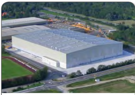
Opening of the assembly building for material handling machines
