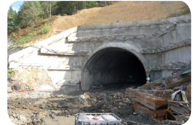
Tunnel driving, Roof, Face & Rib scaling, Floor levelling
