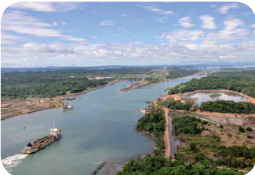
Dock deepening & extension
