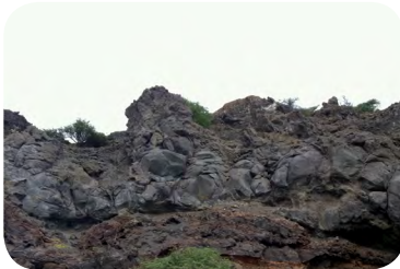
Boulder reduction in rock piles
