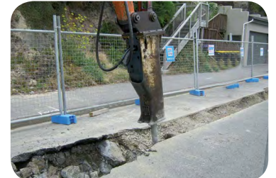
Trenching, pit building, ground excavation
