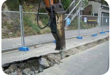
Trenching, pit building, ground excavation
