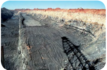
Overburden removal, bench, road & ramp levelling
