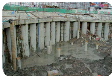
Foundation pile driving
