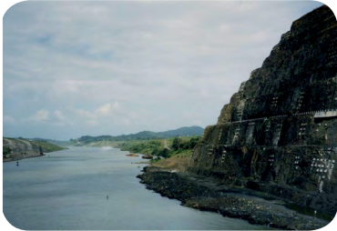
Canal deepening & extension
