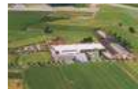
Expanding the production facility in Achtmaal
