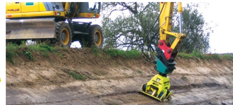
Complicated compaction works on steep slopes and embankments are easily possible
