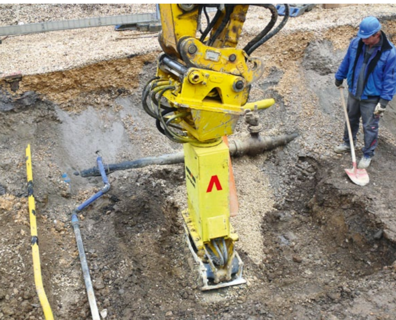
ACA 350-RE with extended upper part used in deep trenches
