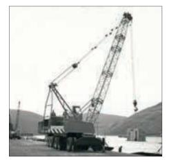
1964: SK 20 cable-operated port crane during cargo handling
